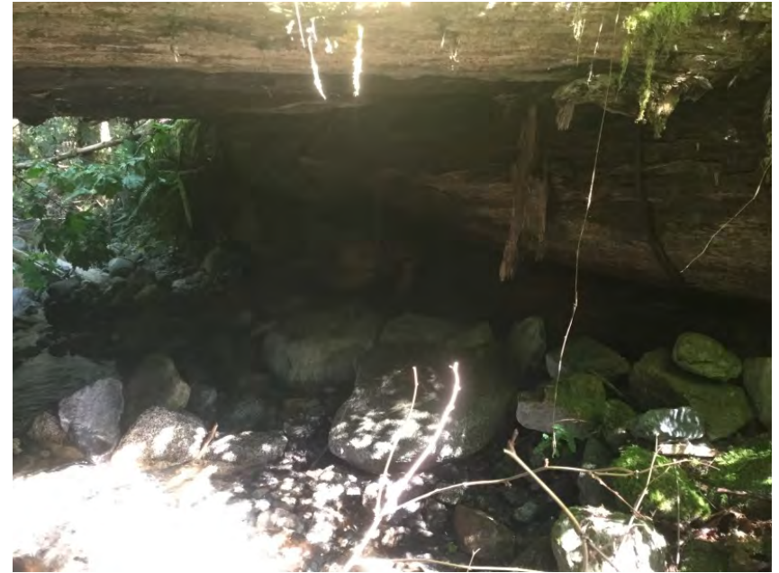
Right Bank Abutment when facing downstream
