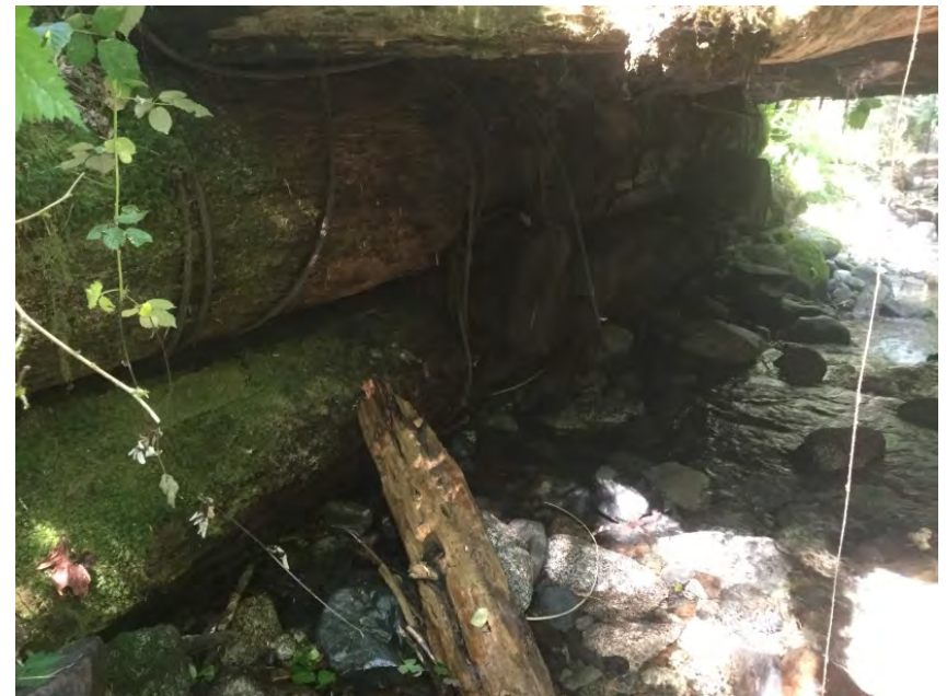
Left Bank Abutment when facing downstream
